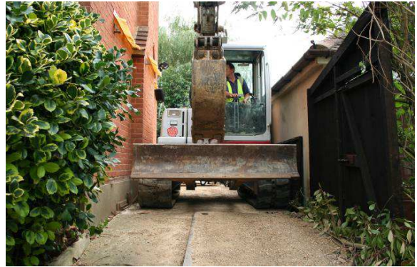
Fig 2 – Machinery appropriate to the site space is utilised.
